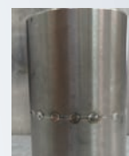
Pipe butt weld Ø 31.75 x 2 mm
